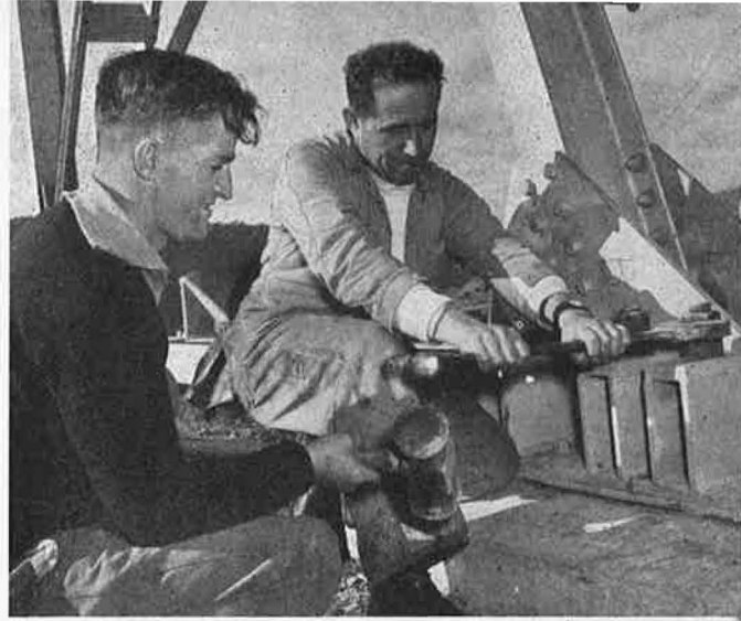
Bolted down. Tom Curtin, front end loader driver, and Harry Austin, heavy driver (with hammer), check the bolts at the base of Pinninger tower. Below:— L: Norm. Collett, linesman, carrying up a dead end. R: Leading hand Hec. Johansen, 20 years in the job.
