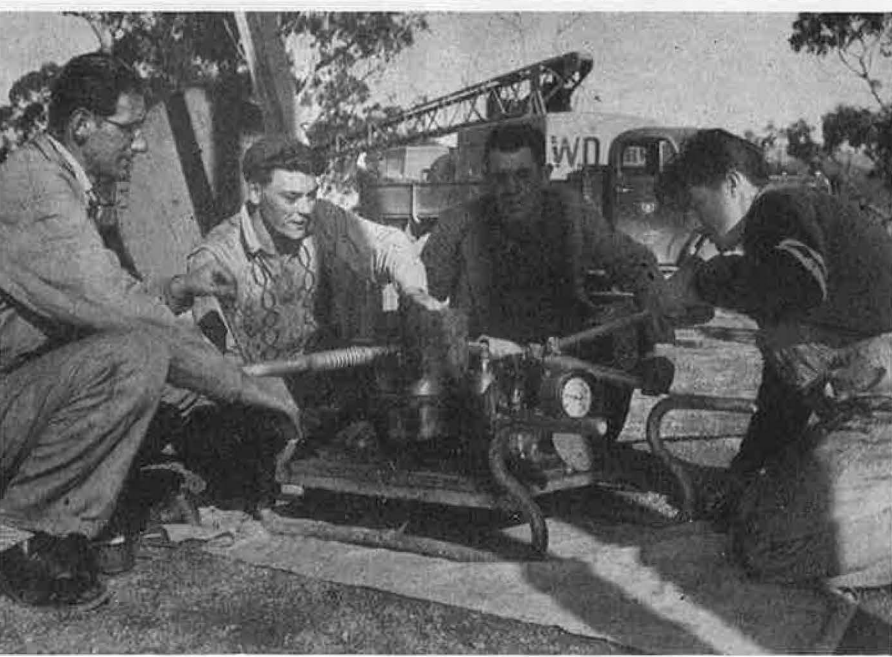
Above: Transmission tower, Mt. Enterprise. Two cables are hooked in. Below: Pressing a dead end on the conductor. From left: R. T. "Lofty" Knight, Tony Biocco, George Fowler, Howard McMahon, working in shadow of Mt. Pinninger transmission tower.
