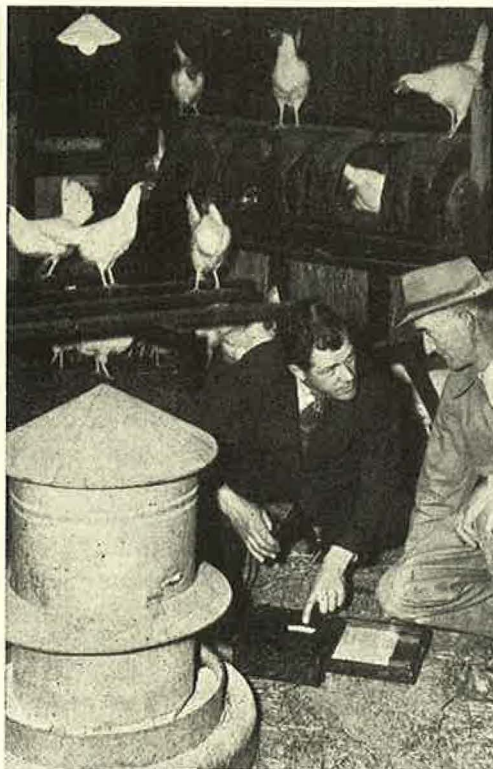
How bright do they like it? Ted Green, rural engineer (L), helps a St. Albans poultry man by measuring intensity of light in this pen.
